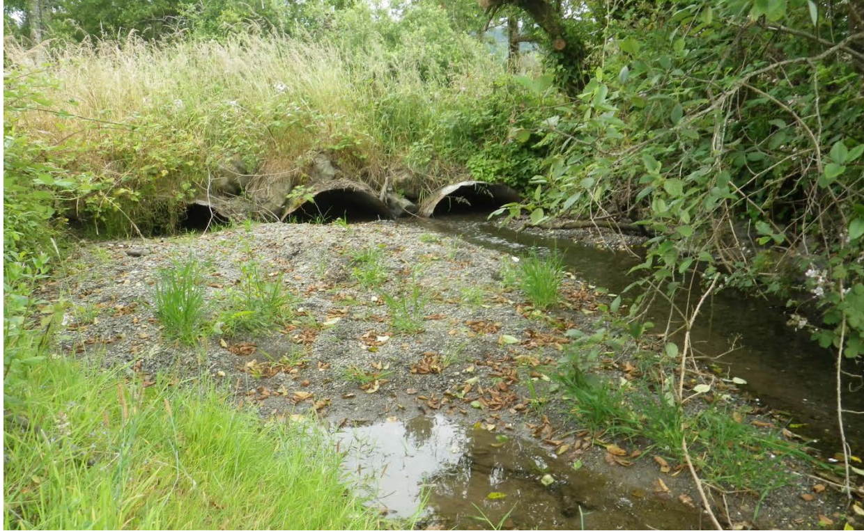
Figure 15. Fred Haight Drive crossing on Morrison Creek. Photo taken on July 17 th , 2012. Note the three 48-inch diameter culverts are almost entirely filled with stream sediments. Flow separations associated with an abrupt bend in the channel upstream of the road, coupled with three separate water paths in the culverts, cause excessive sediment to collect at the crossing increasing localized flooding. Photo: M. Larson
