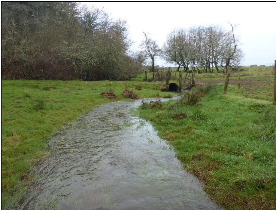
Figure 2-7. 30-inch culverted low-water crossing near the downstream limits of Reach 2 (looking downstream). (January 2020).
