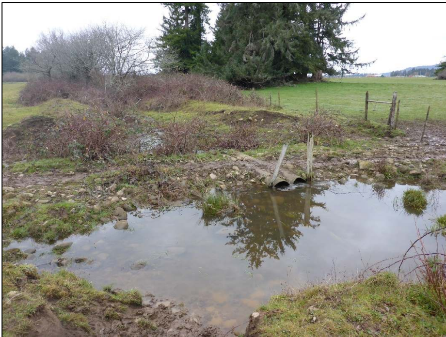
Figure 2-4. Livestock crossing upstream of Lake Earl Drive (looking downstream) consisting of two 18-inch concrete pipes surrounded by placed cobble. (Photo date January 2020).
