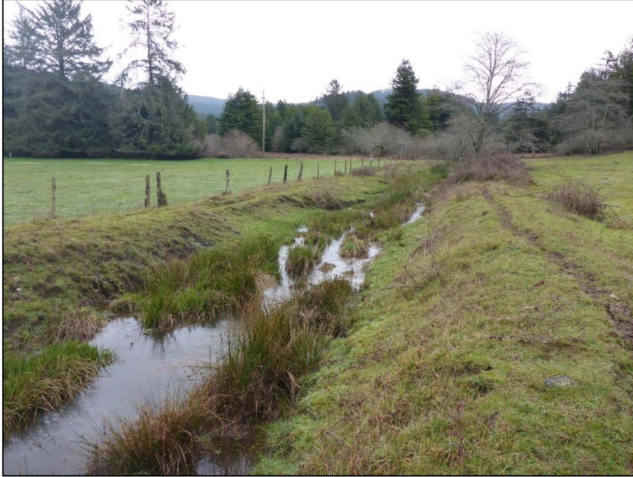
Figure 2-3. Tryon Creek project reach upstream of Lake Earl Drive (looking upstream). The stream channel has been ditched and straightened, with discontinuous spoil piles on both sides of the channel (Photo date January 2020).
