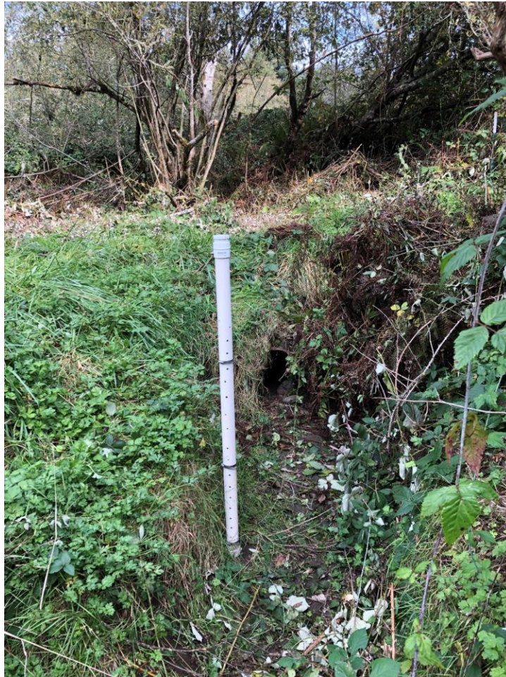
Figure 2-10. View looking upstream at Crossing 5 outlet, visible in photo center. Culvert is 2.5 feet in diameter. Water level logger standpipe visible in foreground is approximately 5 feet tall.
