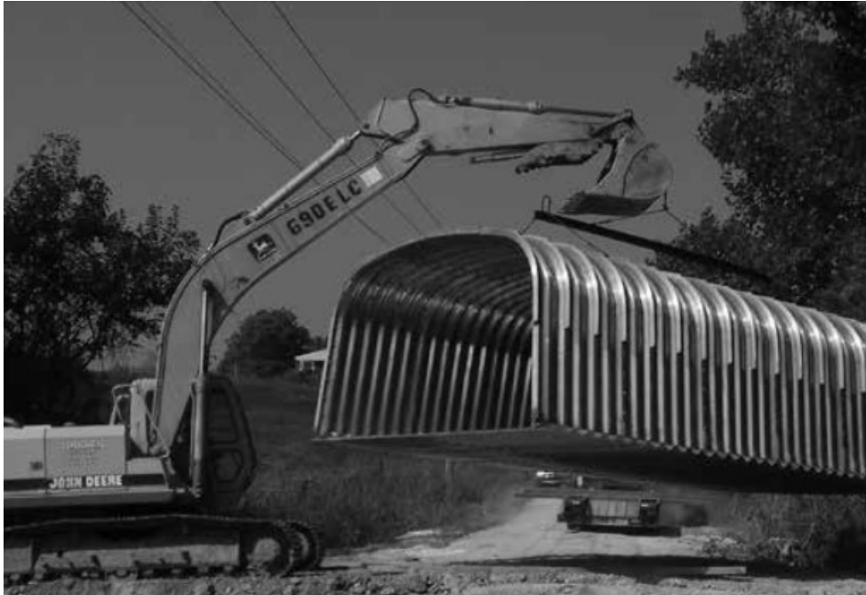
Figure 5-2: Example aluminum box culvert with invert and a plate and rib combination. Photo: Contech
