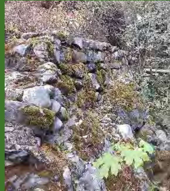
Patrick Creek Historic Structure
